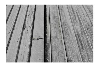
If left untreated, this compromises the coatings on the roofing profile, reducing its life expectancy. As the algae grows and thrives, the top coating begins to breakdown eventually leading to further problems like discoloration, corrosion, and rust.
